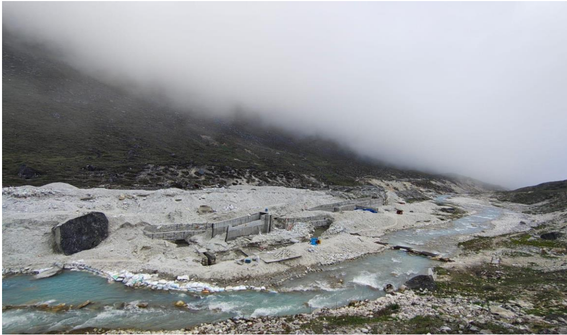
Figure 1: Construction at headworks area
