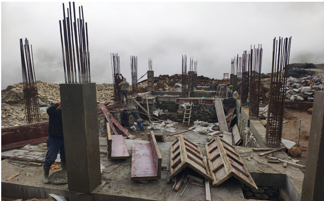
Figure 2: Construction at Powerhouse
