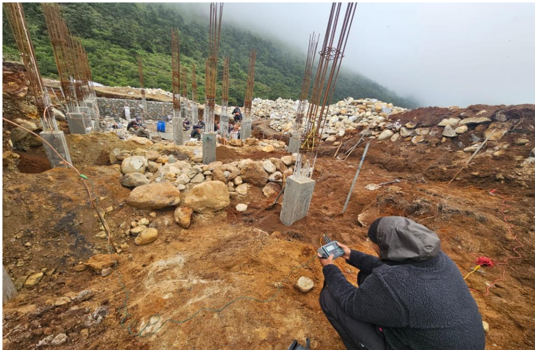
Figure 4: Completion and testing of powerhouse earthing
