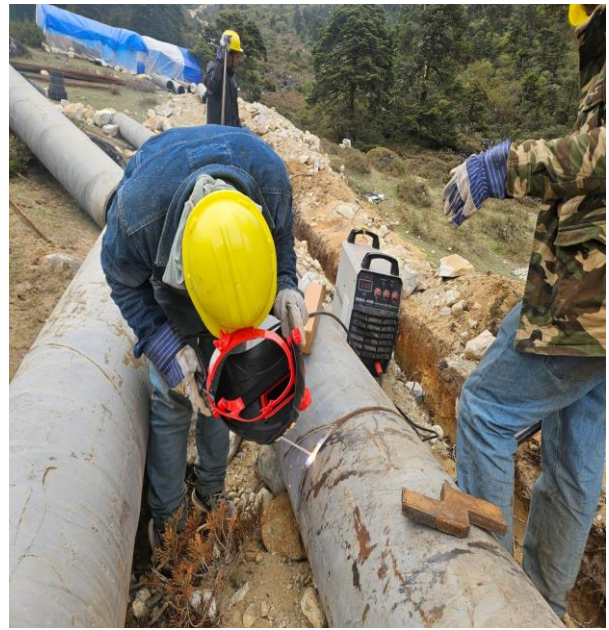
Fig 6. Welding of 15.75mm Penstock Pipe.
