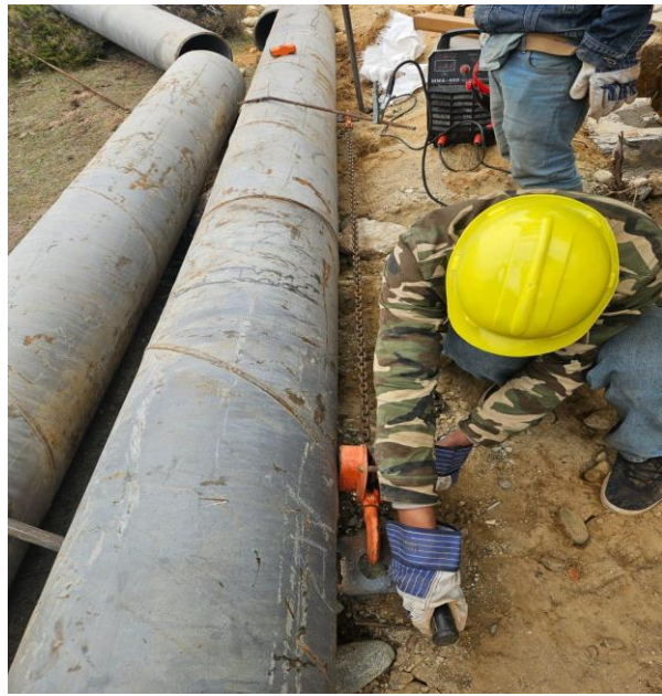
Fig 5. Field Alignment of Penstock Sections
