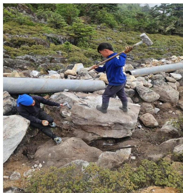
Fig 7. Clearance/Breaking of Boulder encountered at penstock pipe alignment.
