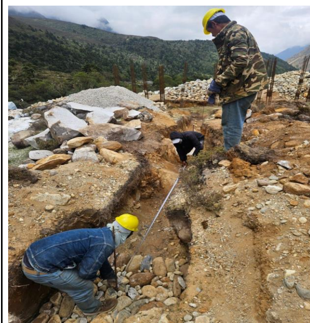
Fig 8. Level check & Penstock length verification at the trench prepared.
