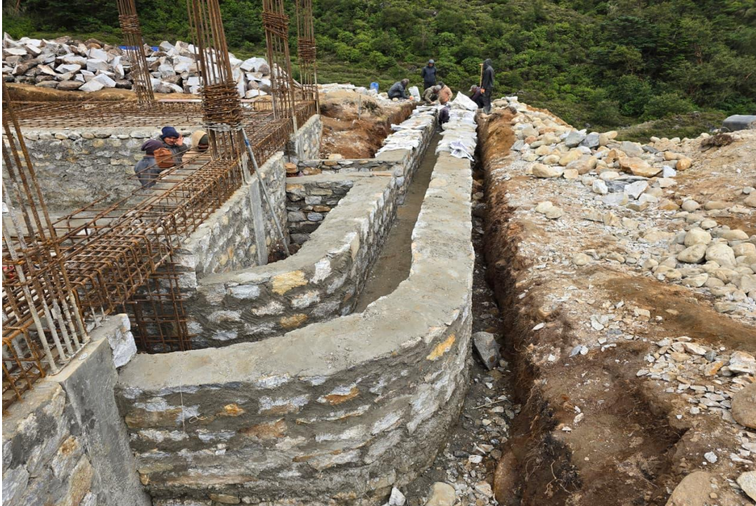
Figure 3: Construction work at powerhouse and tailrace
