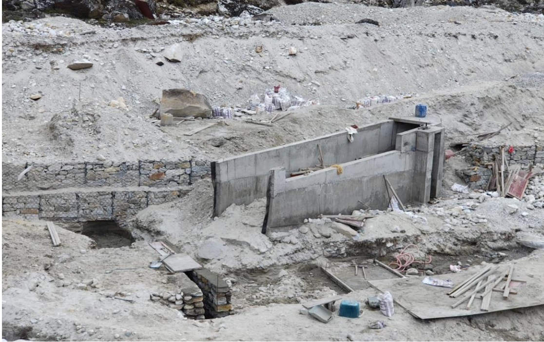
Figure 1 & 2: Construction at headworks area
