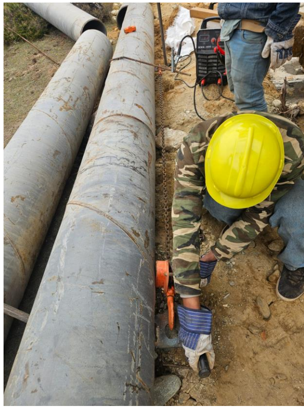
Fig 5. Field Alignment of Penstock Sections Using Chain Puller Before Welding.
