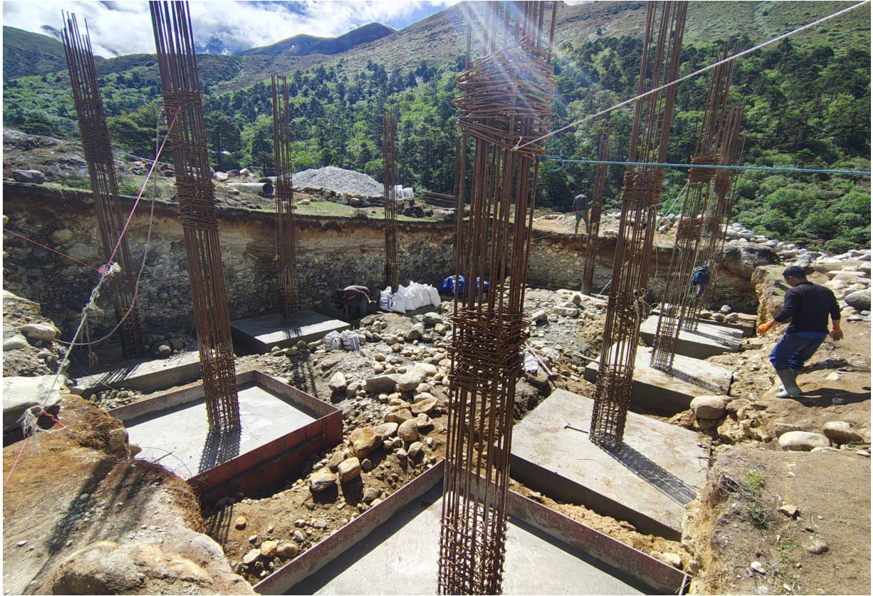
Figure 3: Completion of footing work at powerhouse
