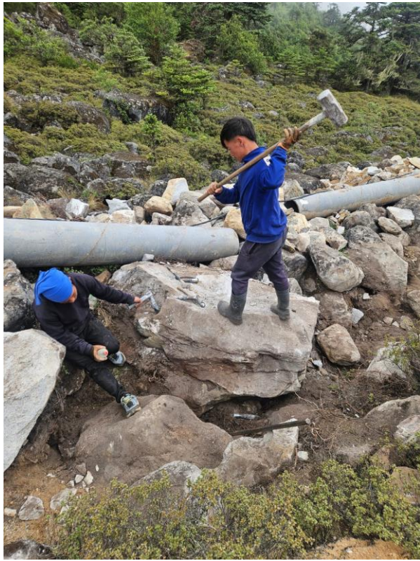
Fig 7. Clearance/Breaking of Boulder encountered at penstock pipe alignment.
