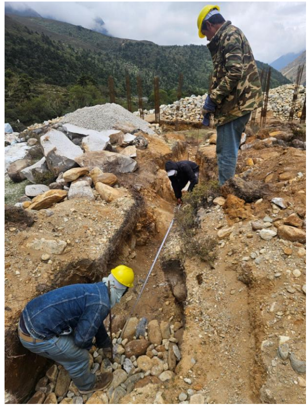
Fig 8. Level check & Penstock length verification at the trench prepared.
