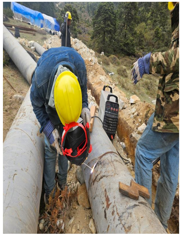
Fig 6. Welding of 15.75mm Penstock Pipe.
