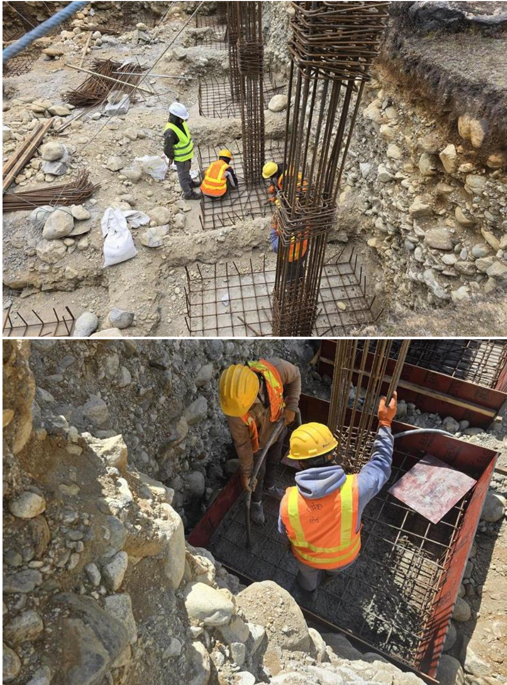
Figure 1 & 2: Preparation for footing of Powerhouse and Concreting works
