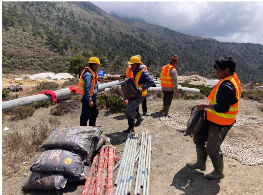
Figure 4: Transportation of Powerhouse Earthing Accessories to site
