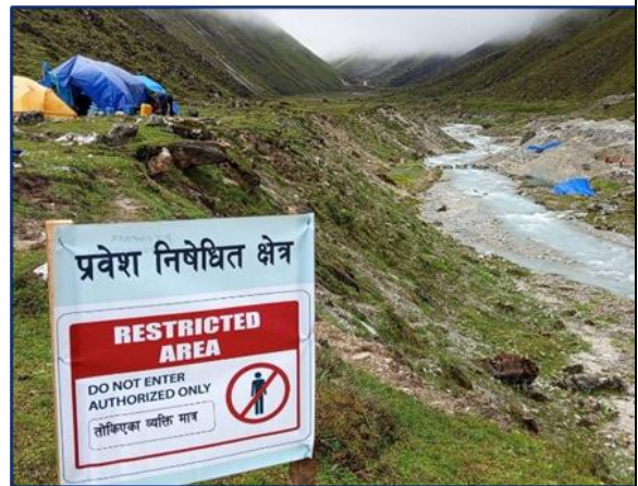
Figure: Existing Construction Signages (Intake)
