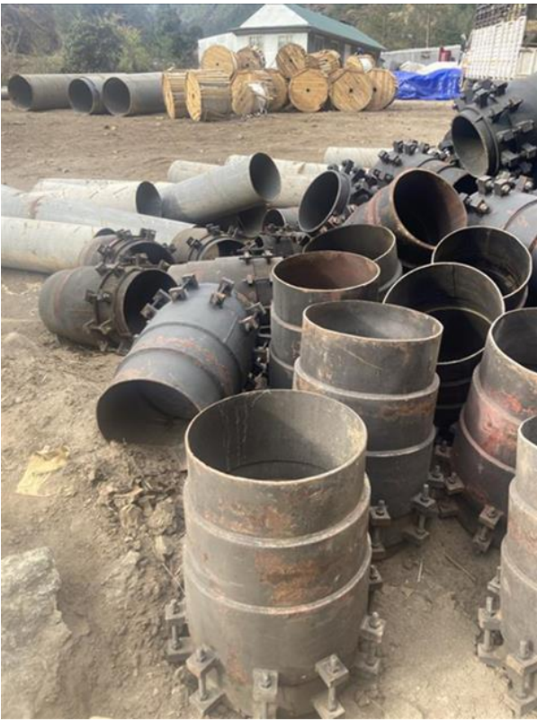
Figure 10 & 11: Bend pipes and expansion joints preparing for airlifting to site
