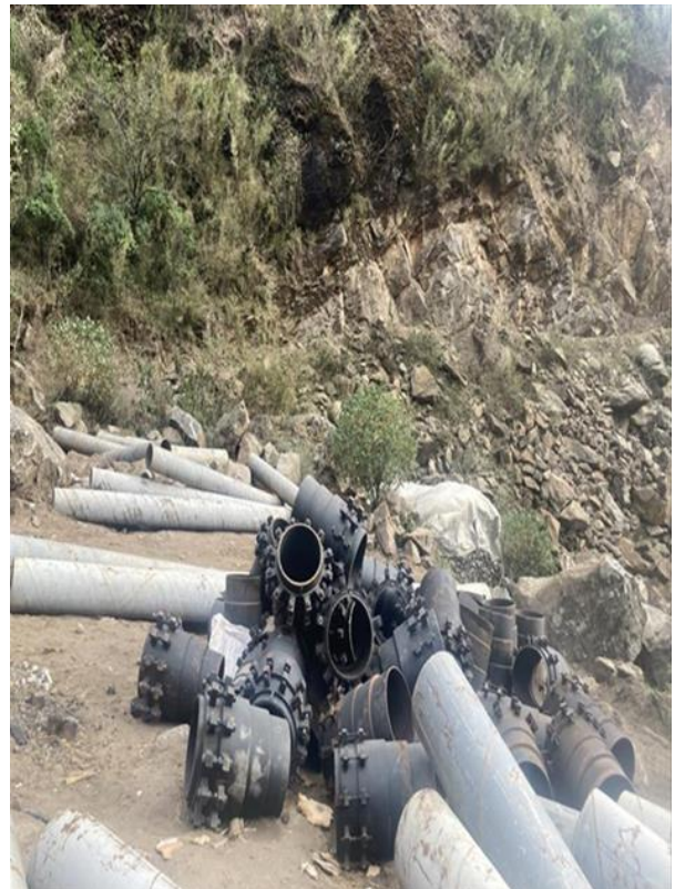
Figure 10 & 11: Bend pipes and expansion joints preparing for airlifting to site
