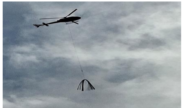
Fig.9: Transportation of Rebar from road head to site
