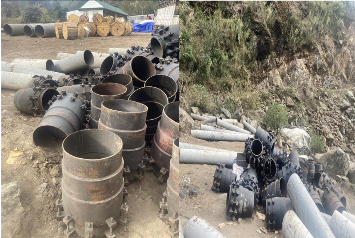
Figure 4 & 5: Bend pipes and expansion joints preparing for airlifting to site
