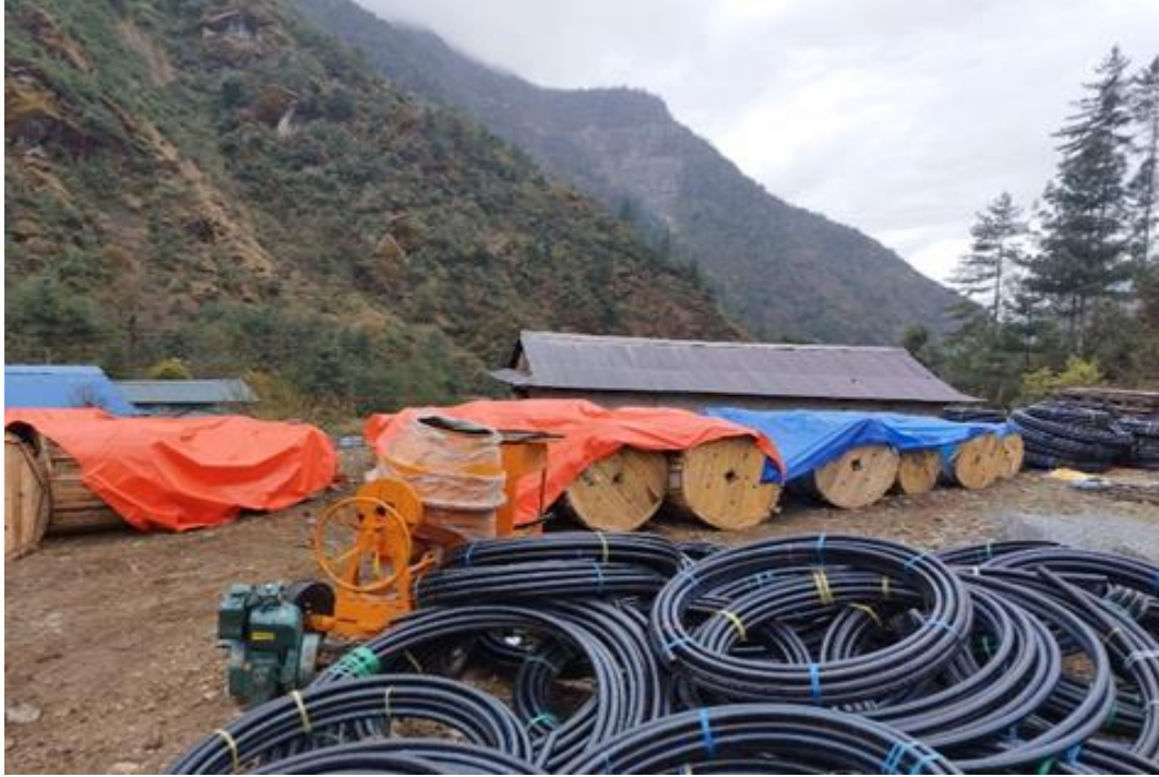
Figure 10: LT cables and service wires prepared for signing as per EDF
