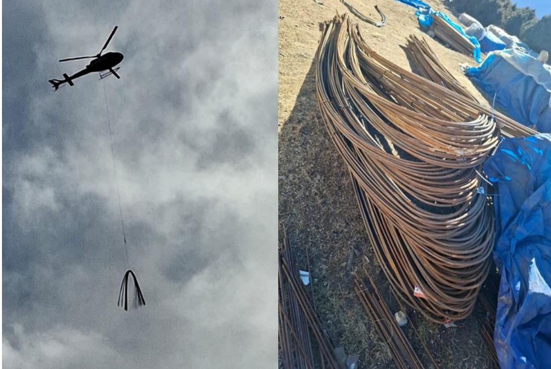
Figure 2&3: Transportation of Rebar from roadhead to site
