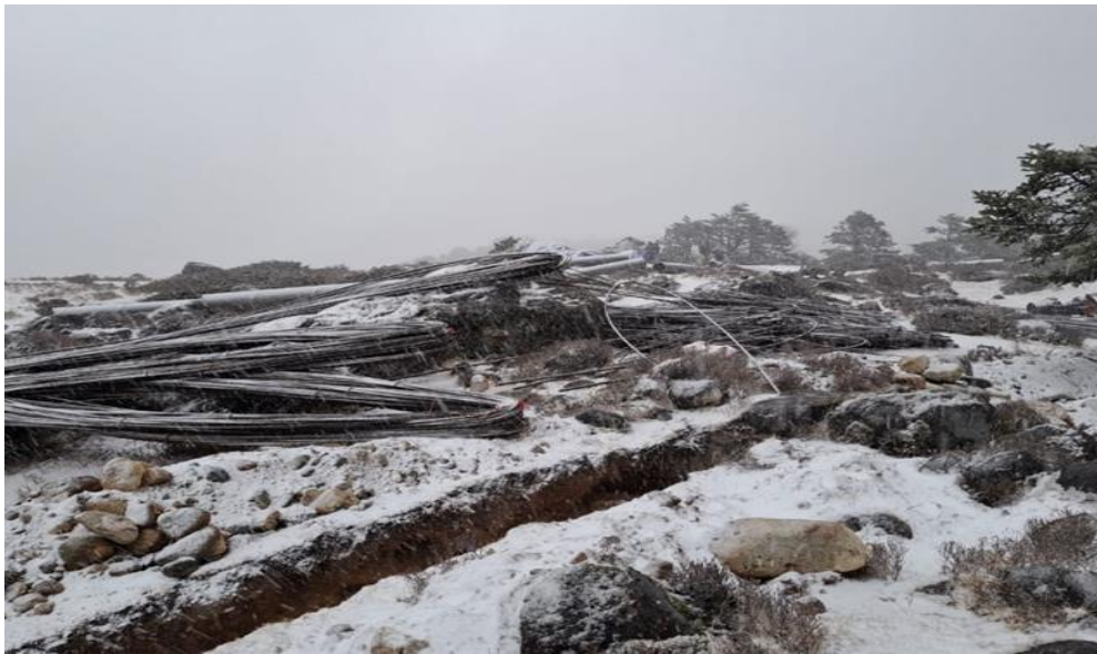
Figure 1: Stacking of Rebar at the project site
