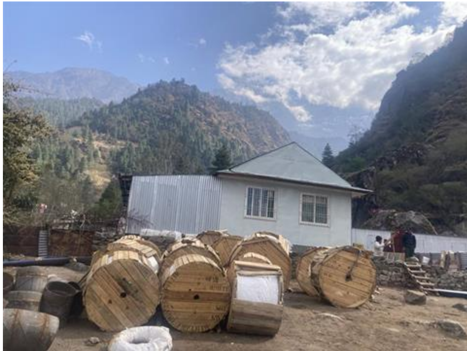
Figure 9: LT cables stored at the roadhead Surke.
