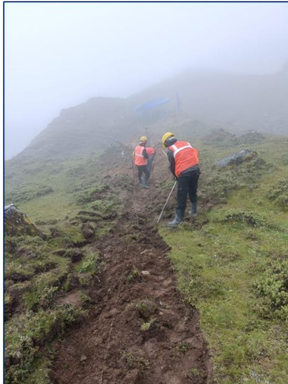
Figure: Topsoil is carefully removed along the pipeline alignment for rehabilitation
