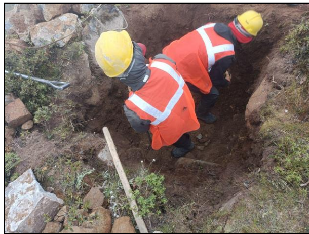
Figure: Labor are working at construction site (Pipeline)
