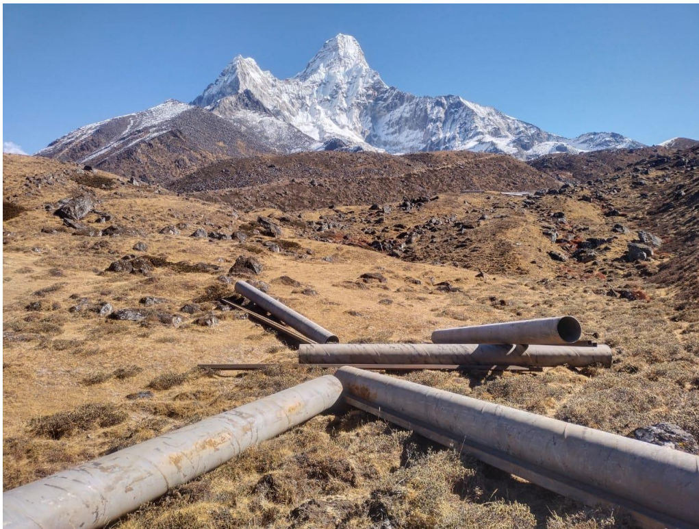
Figure 8 : Pipe dropped by helicopter on the site
