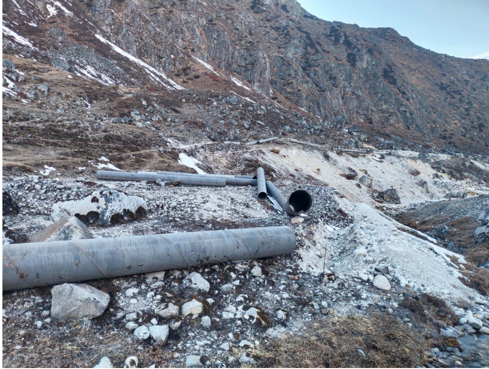
Figure 5: Pipe laying along the penstock alignment
