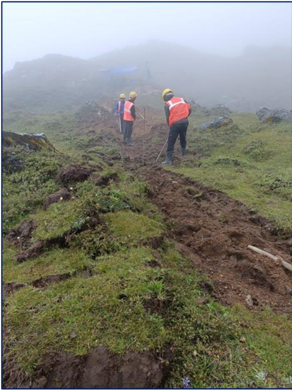
Figure: Topsoil is carefully removed along the pipeline alignment for rehabilitation
