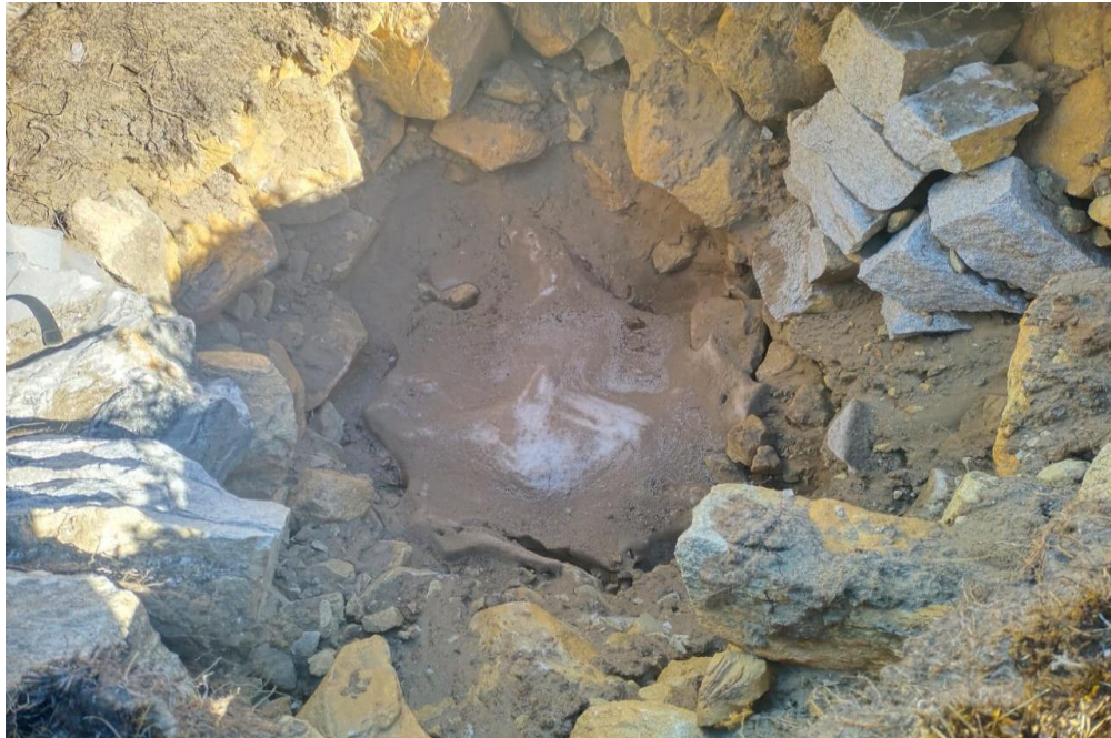
Figure 6: Frozen surface on the excavated anchor block
