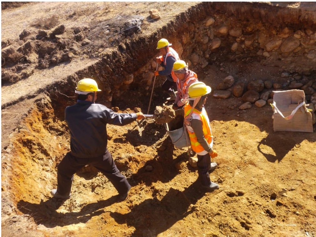
Figure 10 : Excavation works of Powerhouse
