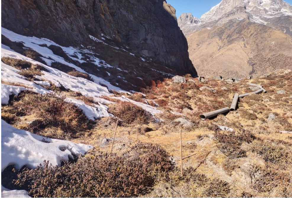
Figure 7: Marking of the anchor block
