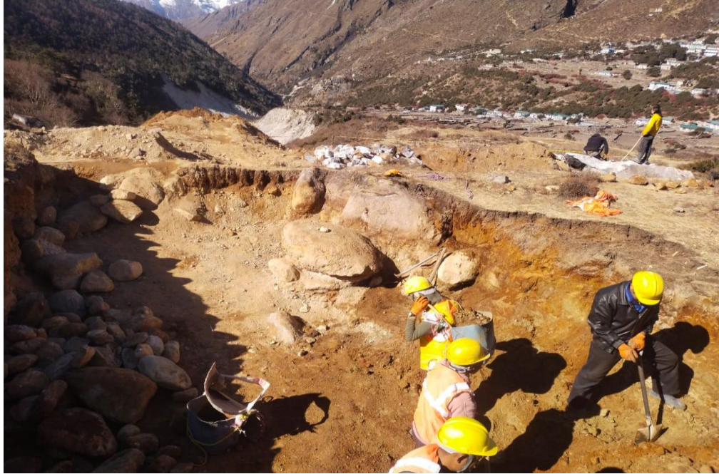
Figure 9 : Excavation works of Powerhouse
