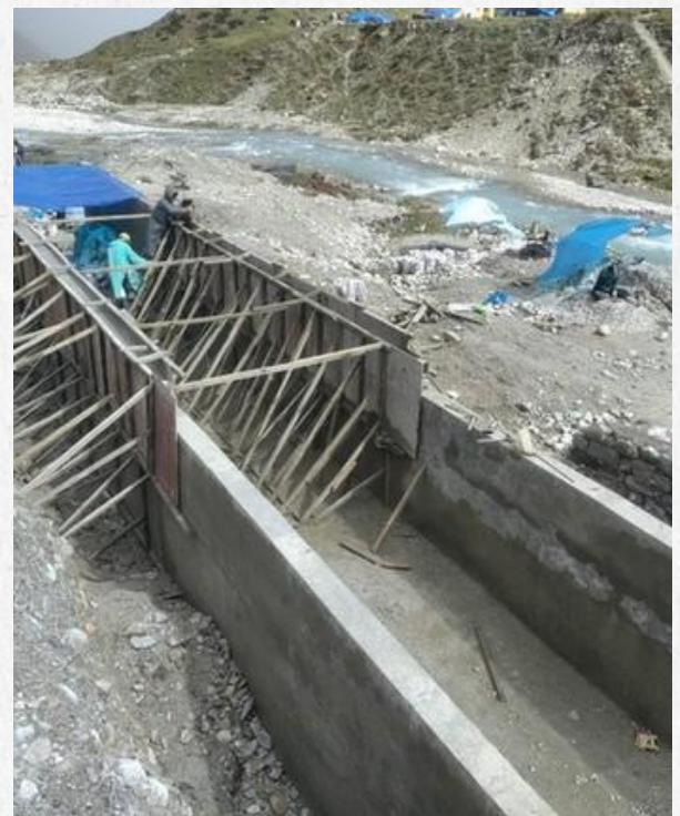
Concreting works of desanding basin
