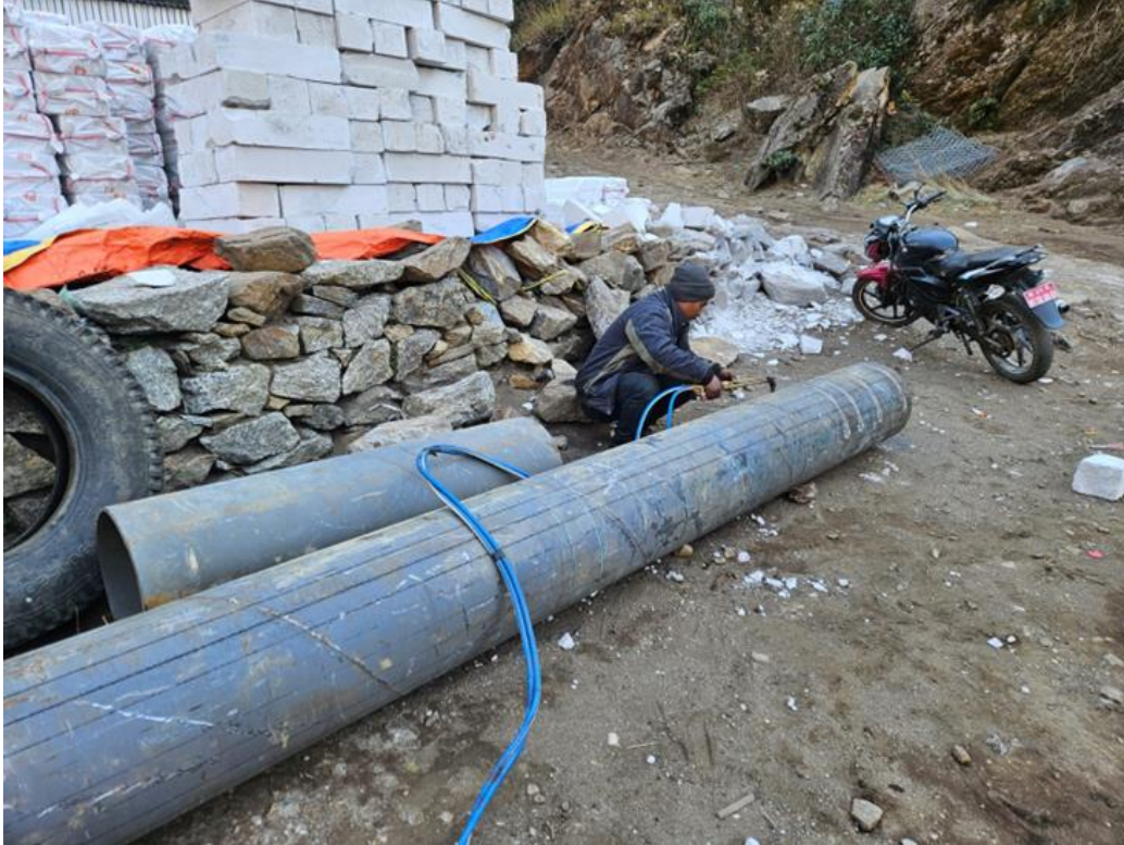
Fig 15. Gas Cutting for Bends
