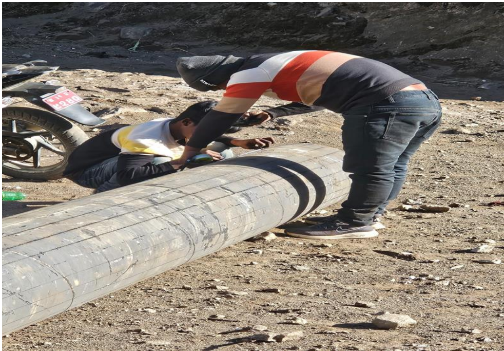
Fig 14. Marking for Bends
