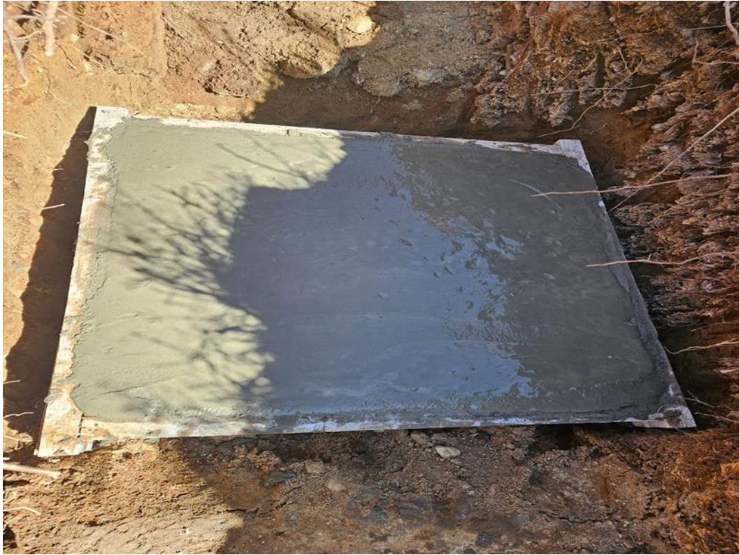
Fig 13. Saddle Support Concrete work
