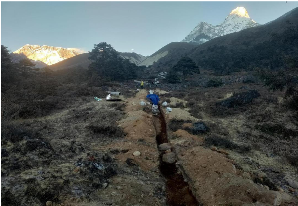
Fig 18. Trench formation for penstock pipe alignment
