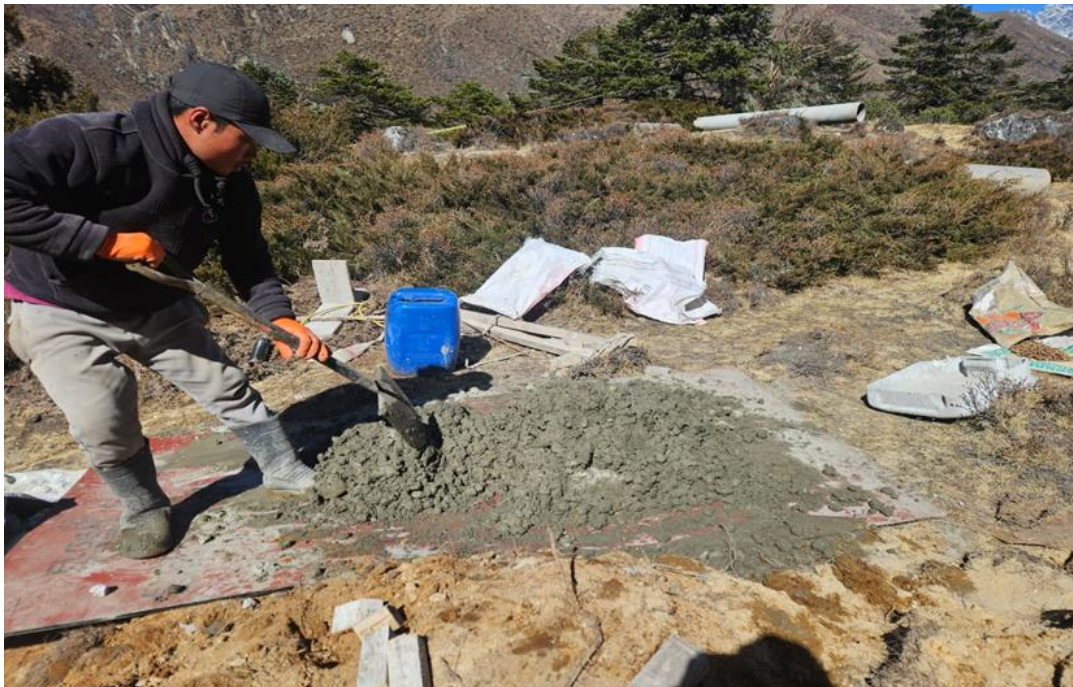
Fig 12. Preparation of concrete for Saddle Support
