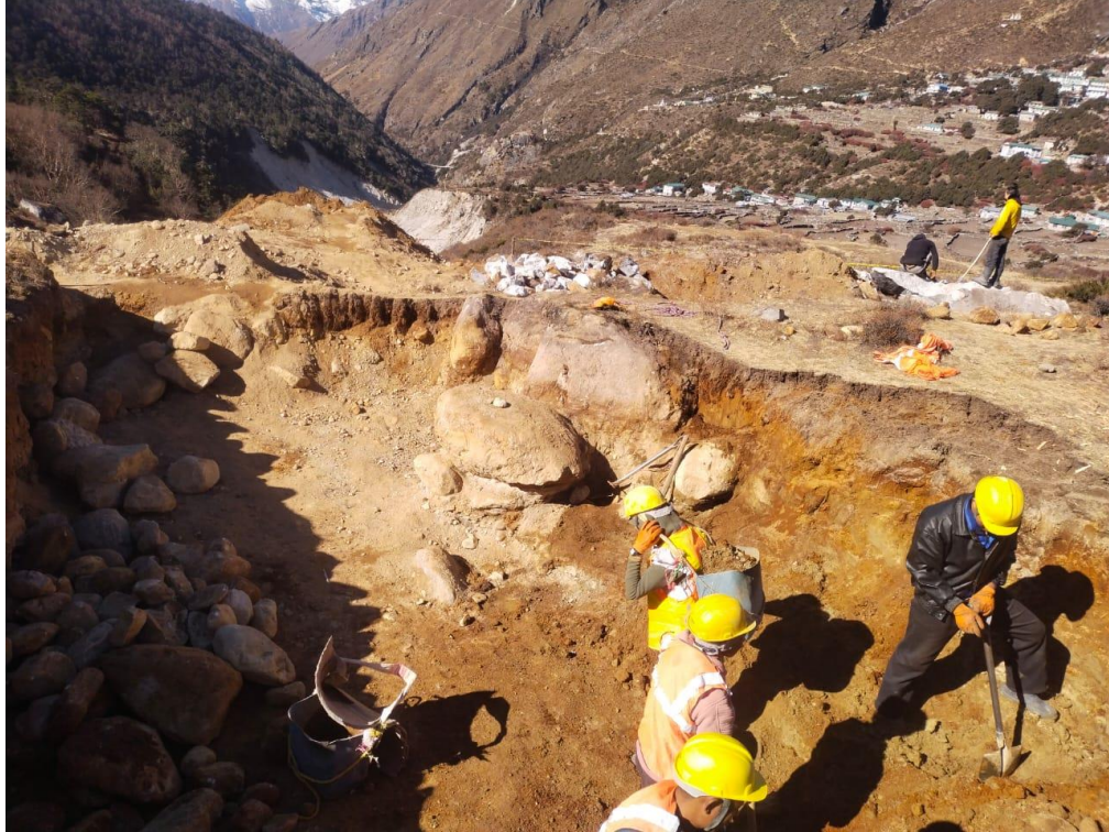
Fig 19. Excavation of Power house area
