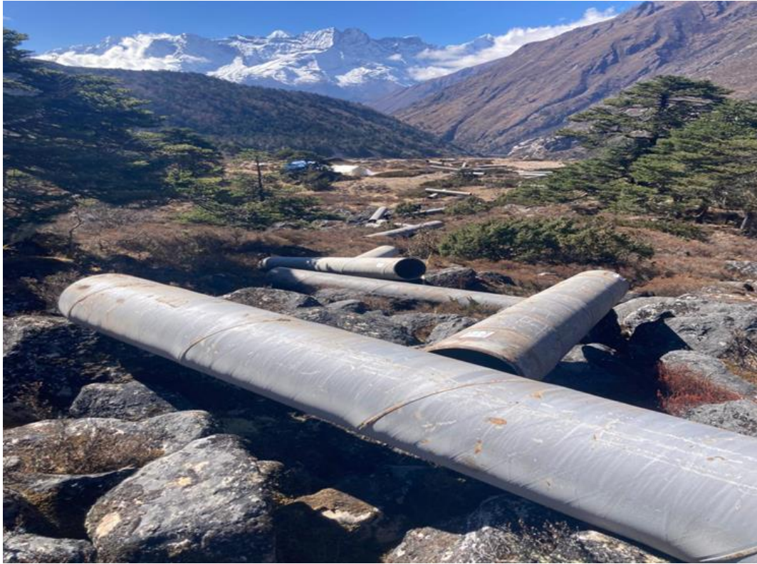
Fig 11. Penstock Pipes being drop at pipe alignment
