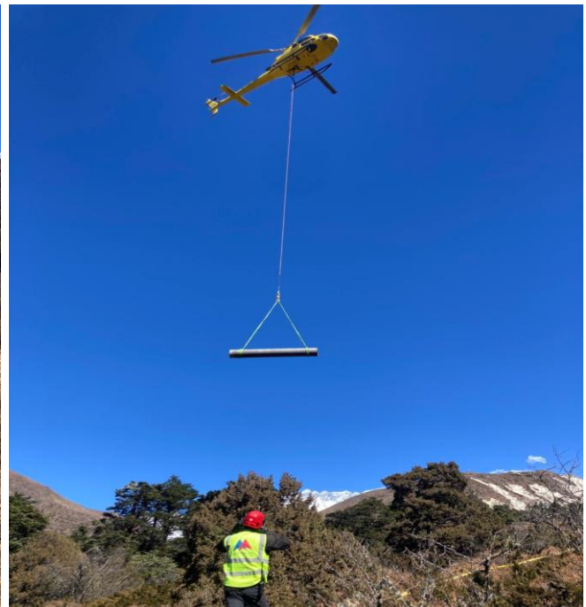
Fig 5. Penstock transportation and alignment at the project site by helicopter
