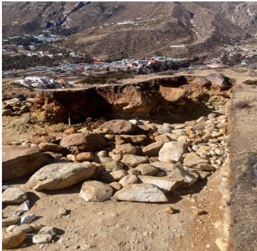
Fig 6. Trench formation for penstock pipe alignment
