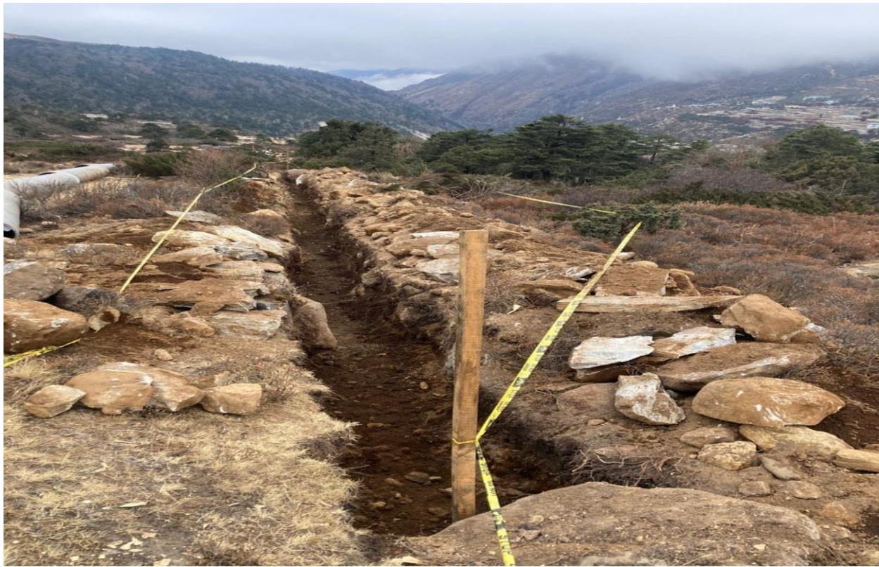
Fig 6. Trench formation for penstock pipe alignment
