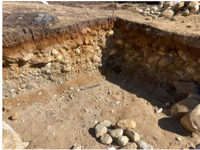
Fig 6. Trench formation for penstock pipe alignment
