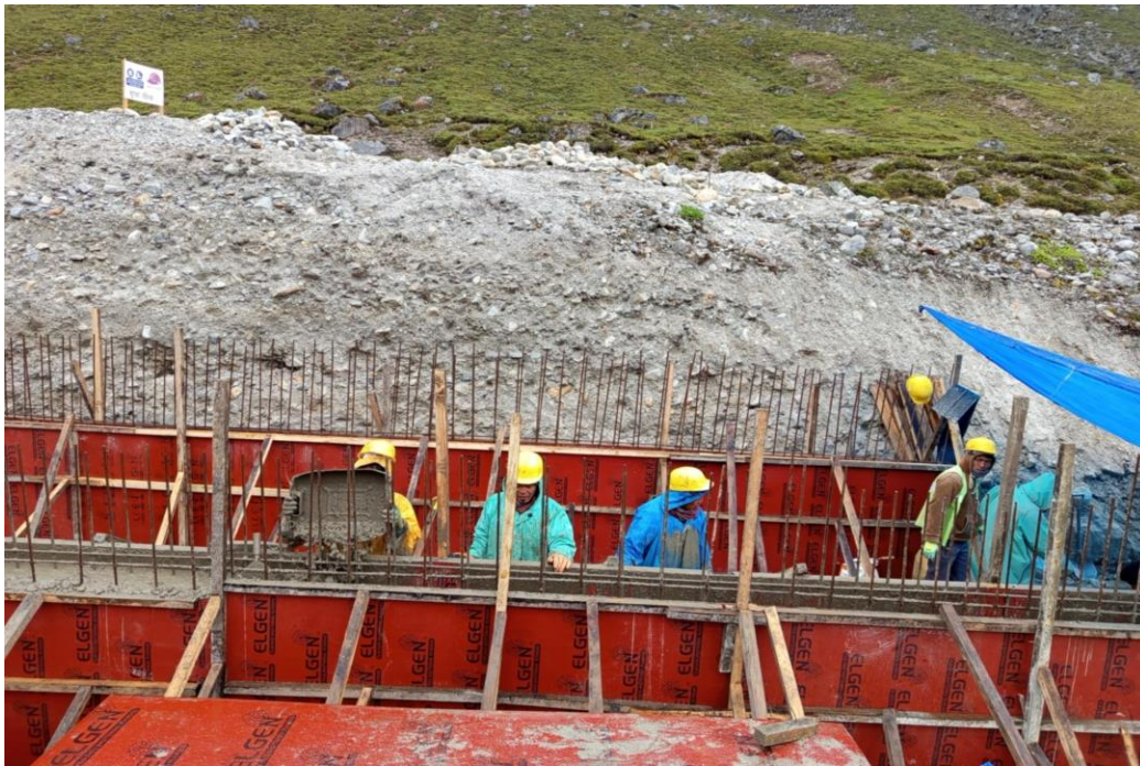
Figure 6: Concreting works in desander basin (Panel 1 - Wall)
