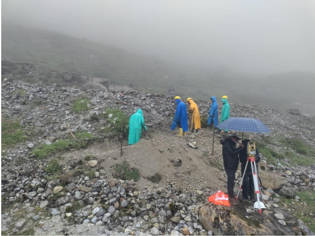
Figure 9: Excavation of Penstock Alignment from Desander Basin to Anchor Block 1
