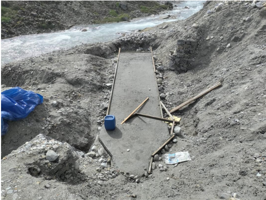
Figure 3: PCC in Gravel Trap
