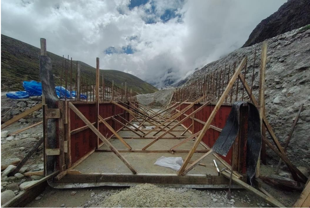
Figure 5: Formworks in Desander Basin wall (Panel 1)
