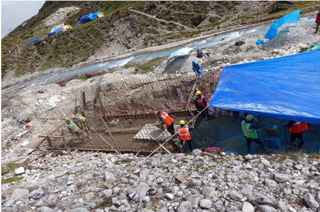
Figure 8: Concreting works in desander basin (Panel 3 - Base)
