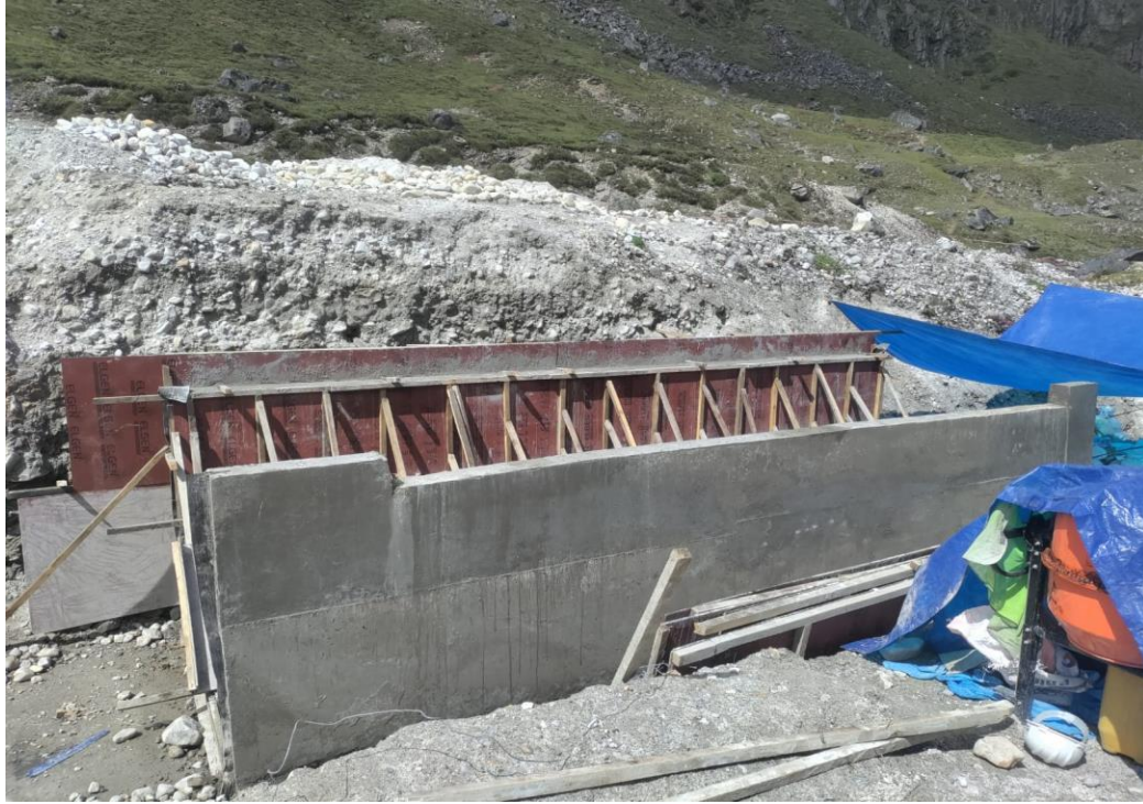
Figure 7: RCC works in desander basin (Panel 1 - Wall)
