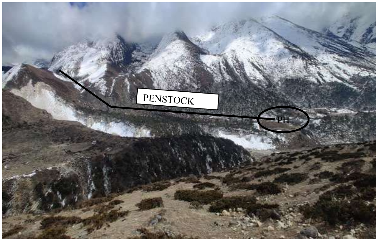
Penstock Alignment and Powerhouse Site
