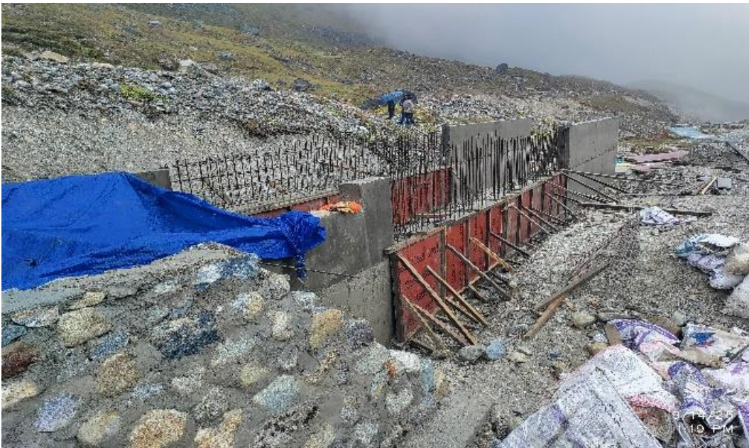
Figure 2: Verge of completion of desander basin
