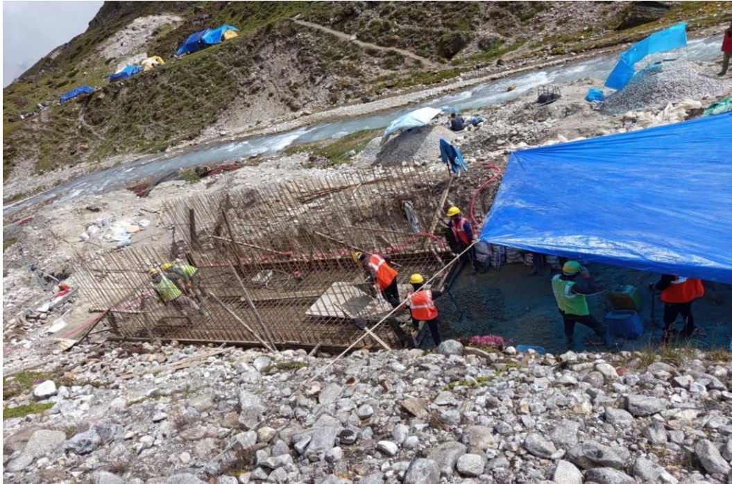
Figure 1: Concreting works in desander basin (Panel 3 - Base)
